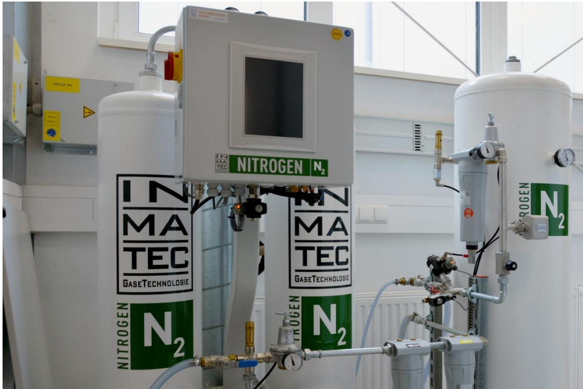
Safety is also a top priority with the protective gas system (nitrogen N2).
